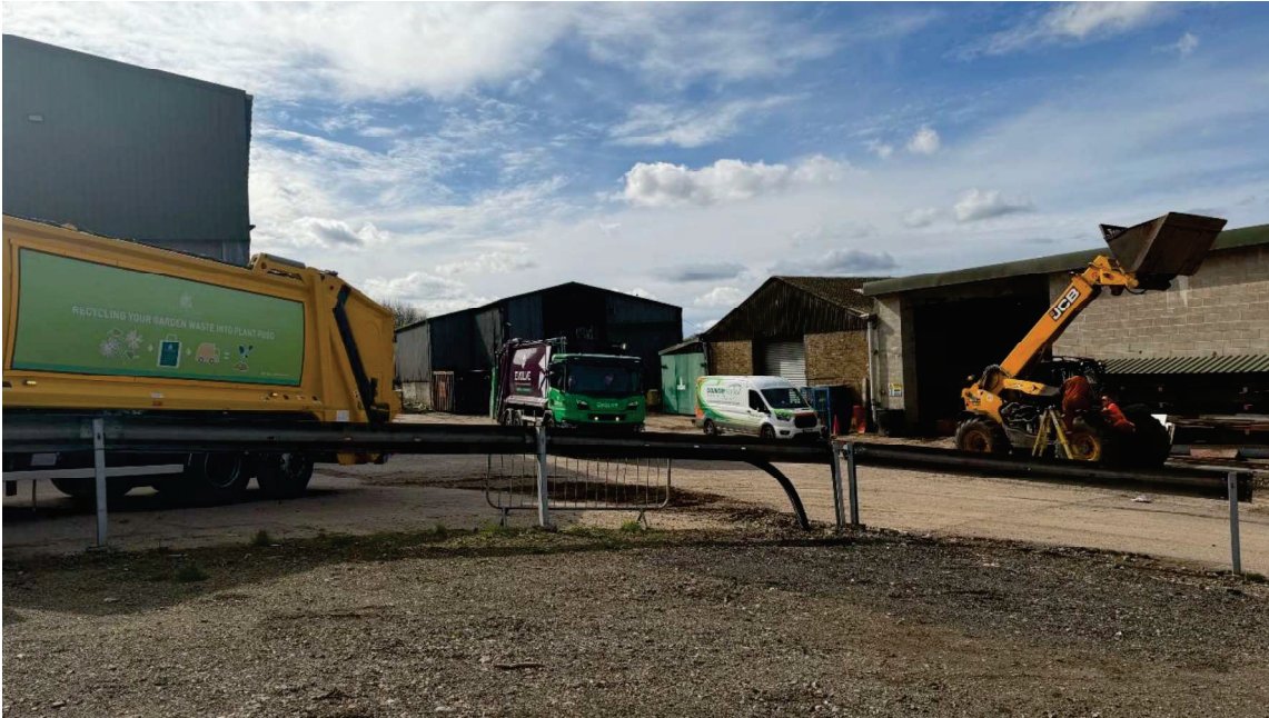
Figure 4: Wider view of existing building within site
